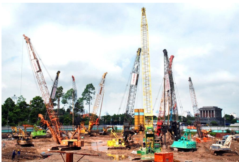
Figure 7: Cast-in-place pile drilling at the new National Assembly building in Hanoi
