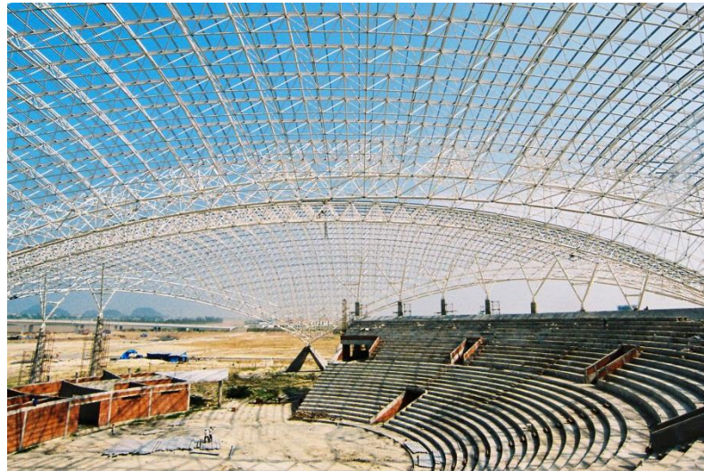
Figure 2: Space frame of Sports hall in Da Nang city
