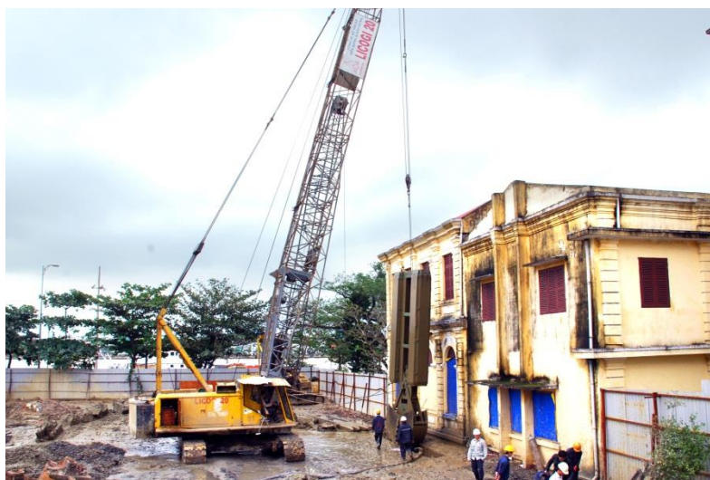
Figure 8: Fence drilling at Han River Hotel – Da Nang
